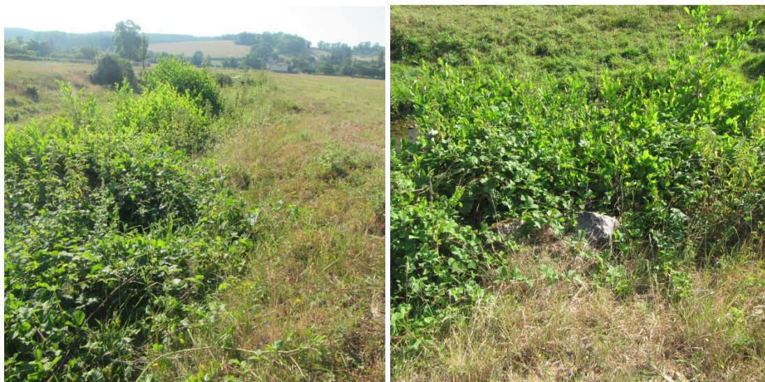
Figure 12 - TH4 : talus amont
