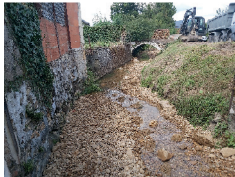
Rivarennas - Le Turpenay amont restauration
